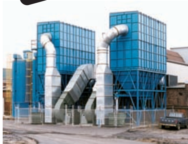
Two TubeJet collectors vent sand handling operations at this foundry. Each collector is rated for 60,000 ACFM.
